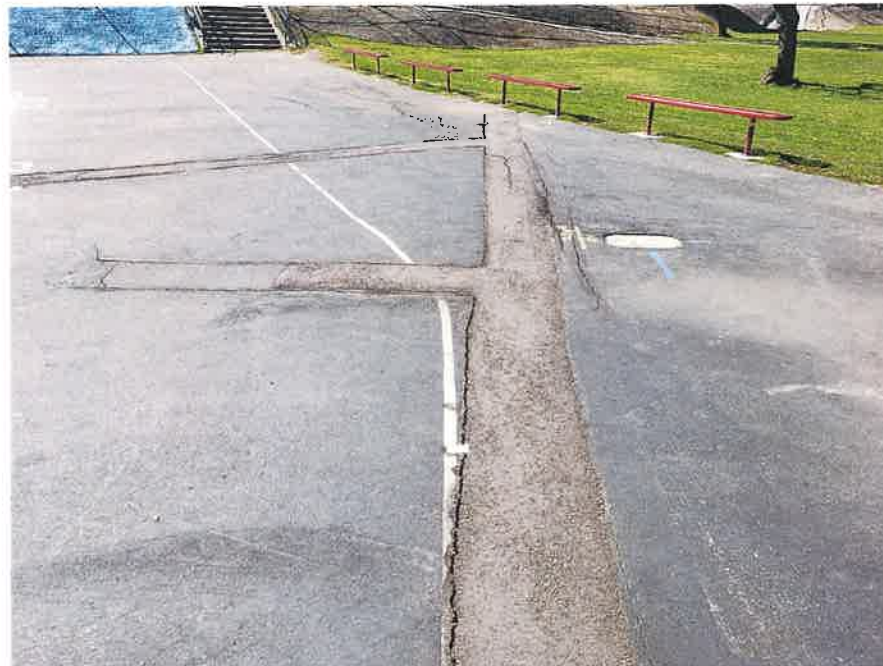
Photograph 4: North Hardcourt: View of play area looking west. Previously patched cracks reopening.
